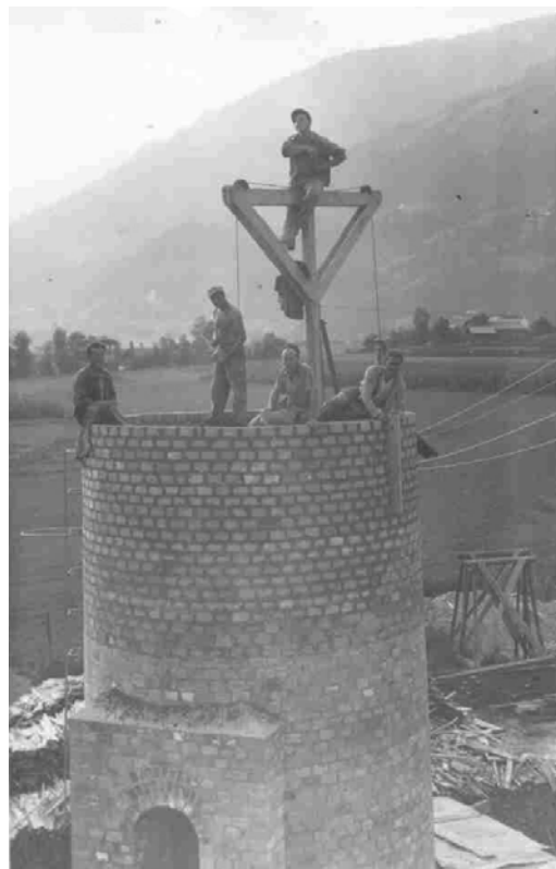
Fig. 1. Furnace masons during chimney construction. Photograph from the collection of FRANZ REINER, now located in the archive of the Museum for Construction Culture at Neutal
